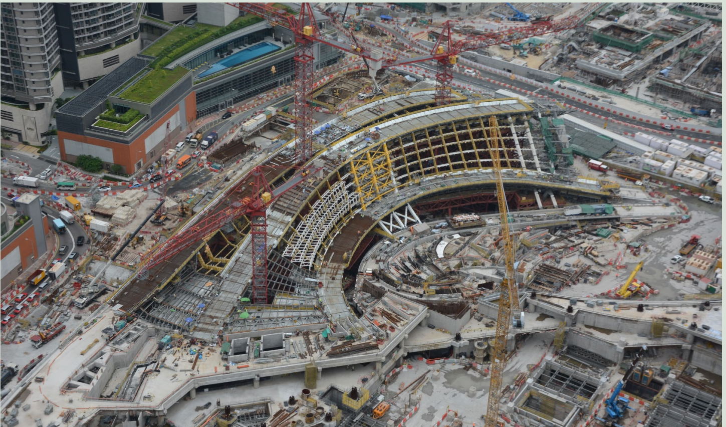
West Kowloon Terminus during construction
