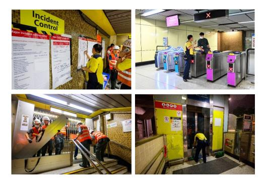
4. Given the unique geographical environment of Entrance/Exit B3 at Wong Tai Sin Station, flood boards have been added in front of the existing flood door to block obstacles that may obstruct the operation of the flood door. A trial on an additional automatic flood barrier will be conducted at the Entrance to explore its feasibility and effectiveness.
